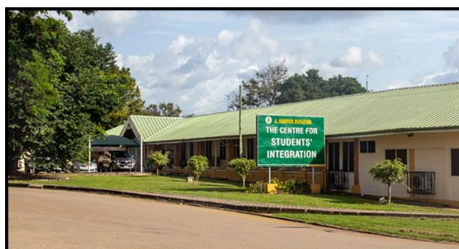
Side View of J Harper Building
